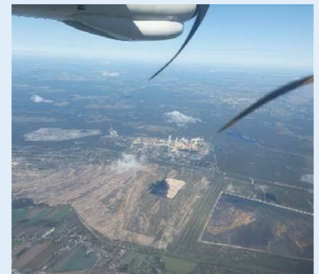
Photo of the Belchatow power plant (Poland) taken on 8 October 2023 from the instrumented aircraft.
