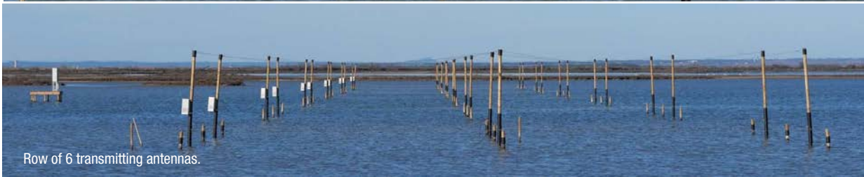
SWR Salins reception antennas with solar panel.
