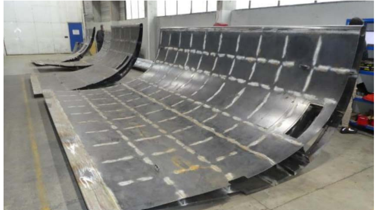
Work to replace the first elbow of the S1MA wind tunnel.
